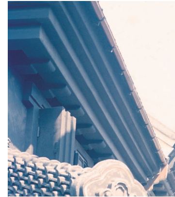
Eave cornice (Fine china store YAMAWA)
