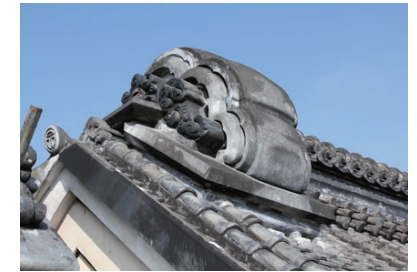
Onigawara decorative tile and kagemori joint (Flagship store of Machikan)
