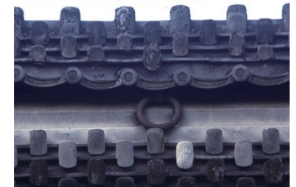
Hakomune roof ridge (Harada House)
