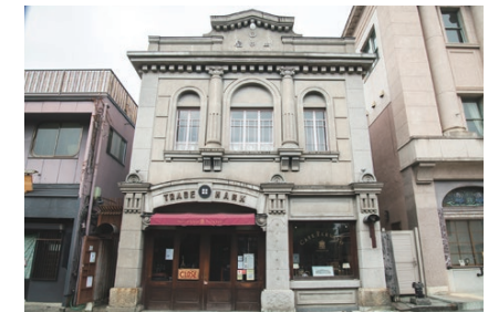
The Former Tanaka Family Residence
